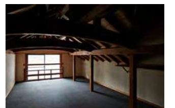
▲ Attic: it uses a traditional Japanese roof framing technique called wagoya.
